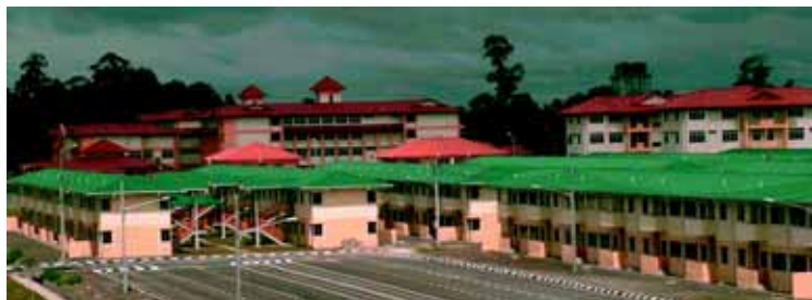
Housing project in Sibujaya, Sarawak.
